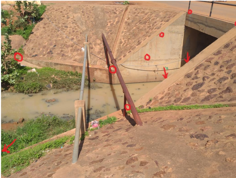
Figure 4 Mesurement points of the structure
